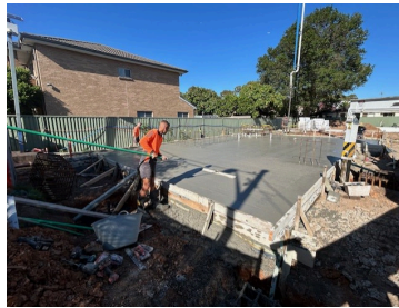
Photo of foundation slab being laid last Monday
